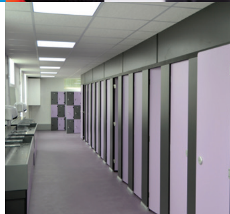
Washroom refurbishments Hayesfield Girls' School, Bath
